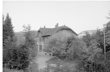
Logement patronal. Phot. Laurent Poupard IVR43_19913900999Z
