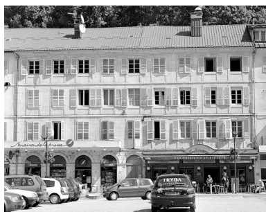
Elévation antérieure. Phot. Yves Sancey IVR43_20033900304X
