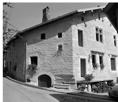
Façade postérieure. Phot. Yves Sancey IVR43_19802500984X
