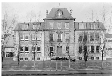
Façade principale. Phot. Jérôme Mongreville IVR43_19872501233X
