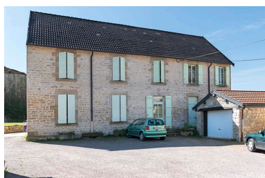
Façade principale. Phot. Sonia Dourlot IVR43_20167000628NUC4A
