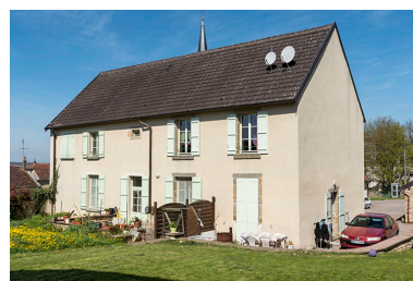
Façade postérieure. Phot. Sonia Dourlot IVR43_20167000629NUC4A
