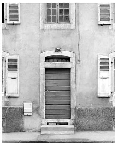
Entrée principale. Phot. Yves Sancey IVR43_20033900467X
