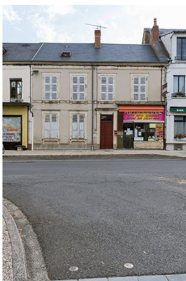
Façade, vue de face. Phot. Pierre-Marie Barbe-Richaud IVR26_20205800573NUC4A
