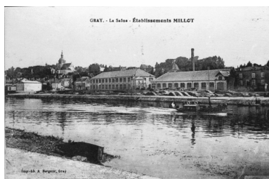
Gray.- La Saône. Etablissement Millot. Phot. Yves Sancey IVR43_19857000116V
