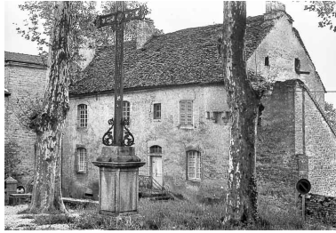
Vue de situation. Phot. Guy Forestier IVR43_19743900738Z
