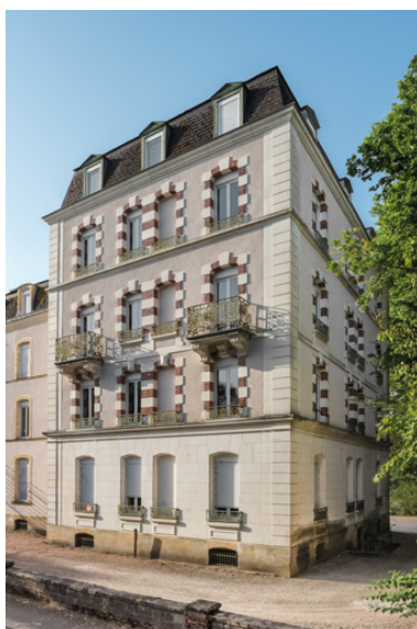
Pavillon occidental. Phot. Pierre-Marie Barbe-Richaud IVR26_20195800549NUC4A
