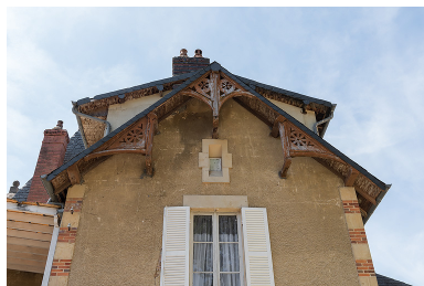
Pignon nord-est. Phot. Pierre-Marie Barbe-Richaud IVR26_20195800672NUC4A
