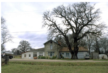
Façade antérieure. Phot. Yves Sancey IVR43_19973900367ZA
