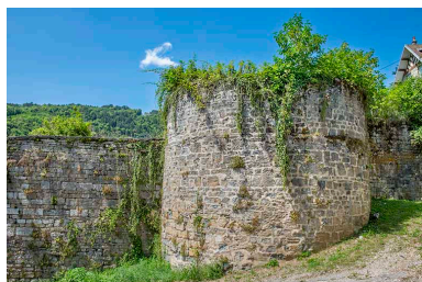
Tour Rouge. Phot. Jérôme Mongreville IVR43_20233900964NUC4A
