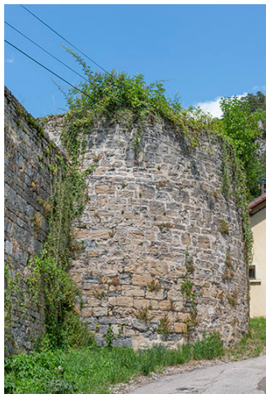
Tour Rouge (front sud). Phot. Jérôme Mongreville IVR43_20233900963NUC4A
