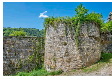
Tour Rouge. Phot. Jérôme Mongreville IVR43_20233900964NUC4A
