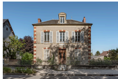
Façade principale. Phot. Pierre-Marie Barbe-Richaud IVR26_20205800506NUC4A
