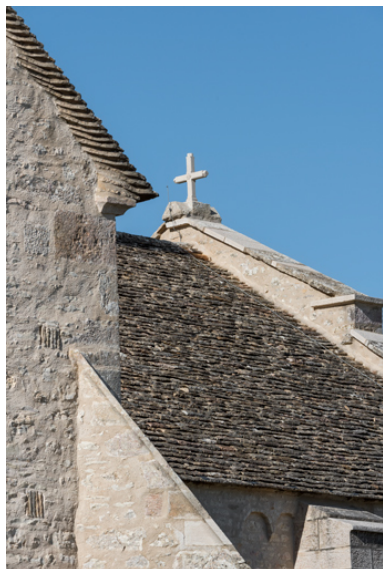
Couverture de la nef. Phot. Pierre-Marie Barbe-Richaud IVR26_20237100293NUC4A
