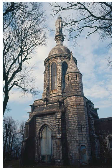
Façade. Phot. Jean-Luc Duthu IVR26_20062106775ZA
