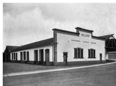
Ateliers divers. Phot. Raphaël Favereaux, Autr. IVR43_20122501352NUC2A
