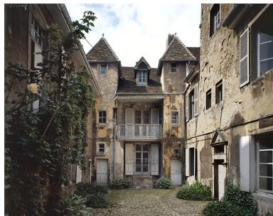
Façade antérieure. Phot. Yves Sancey IVR43_19883900105VA
