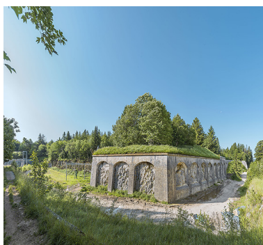
Bastion au front nord. Phot. Thierry Kuntz IVR43_20253900387NUC4A
