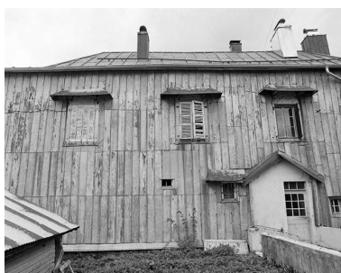
Façade sud. Phot. Yves Sancey IVR43_19993900249X
