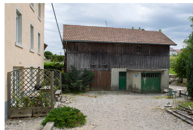
Garage. Phot. Sonia Dourlot IVR43_20142501775NUC2A
