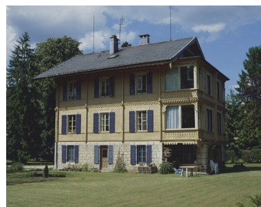
Chalet. Façade sud. Phot. Yves Sancey IVR43_20029000302XA
