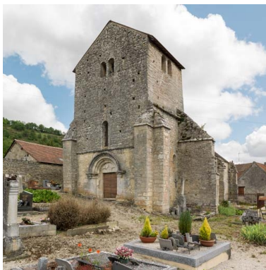
Façade principale. Phot. Pierre-Marie Barbe-Richaud IVR26_20182100116NUC2A
