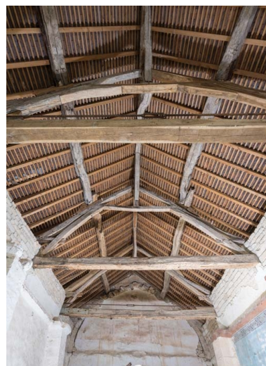
La charpente de la nef. Phot. Pierre-Marie Barbe-Richaud IVR26_20182100075NUC4A
