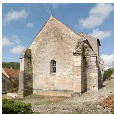
Chevet. Phot. Pierre-Marie Barbe-Richaud IVR26_20182100112NUC2A
