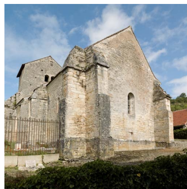
Chevet. Phot. Pierre-Marie Barbe-Richaud IVR26_20182100111NUC2A
