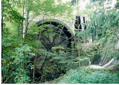
Roue hydraulique verticale. Phot. Laurent Poupard IVR43_19903900454ZA
