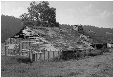
Façade postérieure. Phot. Gilbert Poinot IVR43_19752500941Z
