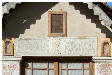
Linteau et niches. Phot. Sonia Dourlot IVR43_20172501801NUC4A
