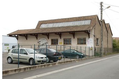
Magasin industriel (?). Phot. Jérôme Mongreville IVR43_20077000675NUCA
