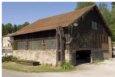
Magasin industriel. Phot. Jérôme Mongreville IVR43_20067000594NUCA
