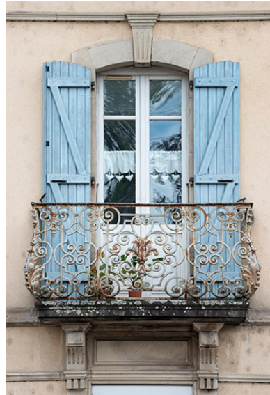
Le balcon, travée centrale. Phot. Jérôme Mongreville IVR43_20177000987NUC4A
