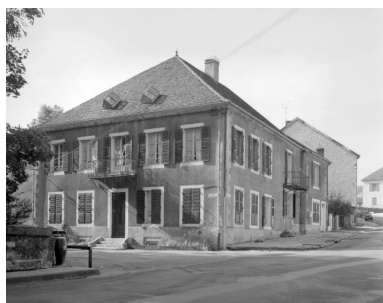
Logement. Phot. Yves Sancey IVR43_19973901326X
