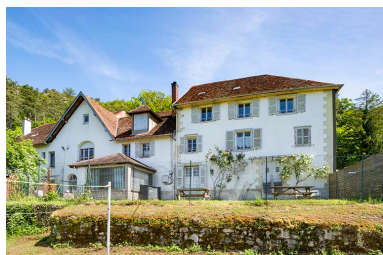
Façades ouest. Phot. Jérôme Mongreville IVR43_20243900687NUC4A
