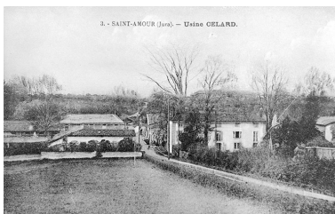
Saint-Amour (Jura).- Usine Célard. Phot. IVR43_19933900395X
