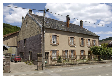
Logement. Phot. Jérôme Mongreville IVR43_20057000362NUCA
