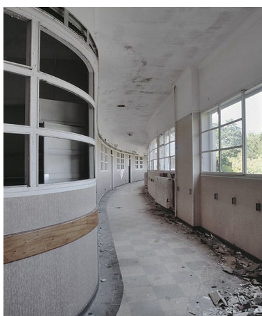
Aile ouest, couloir nord. Phot. Michel Rosso IVR26_20012101234XA
