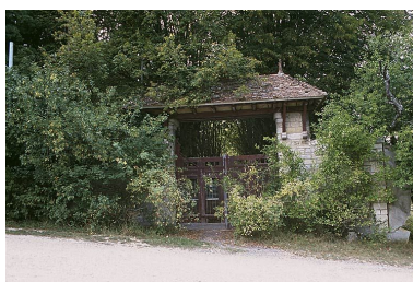
Portail est. Phot. Michel Rosso IVR26_20012101197ZA
