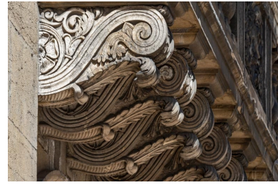
Consoles. Phot. Pierre-Marie Barbe-Richaud IVR26_20222100670NUC4A
