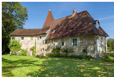
Elévation ouest. Phot. Sonia Dourlot IVR43_20167000816NUC2A
