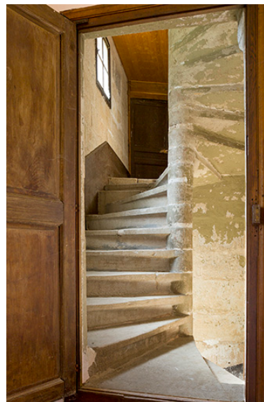
Escalier en vis. Phot. Sonia Dourlot IVR43_20167000820NUC2A
