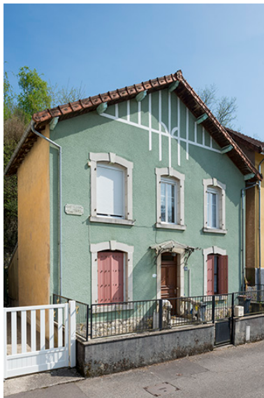
Façade principale. Phot. Jérôme Mongreville IVR43_20177000507NUC4A
