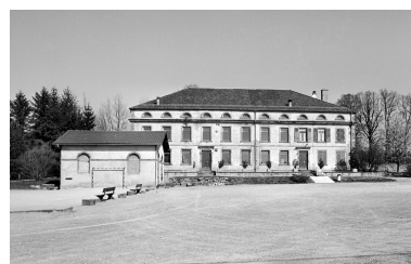
Façades sud. Phot. Yves Sancey IVR43_20039000073X
