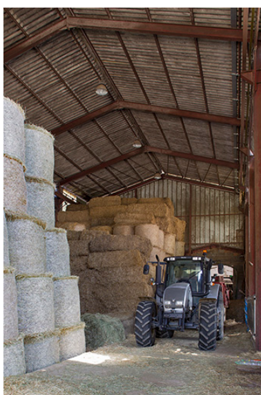
Fenil. Phot. Sonia Dourlot IVR43_20142500992NUC2A
