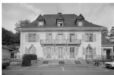
Façade sud. Phot. Jérôme Mongreville IVR43_19872501140V
