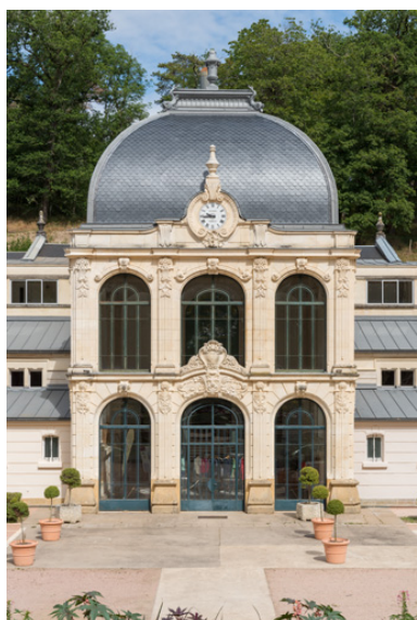
Pavillon central, vue de face. Phot. Pierre-Marie Barbe-Richaud IVR26_20195800409NUC4A
