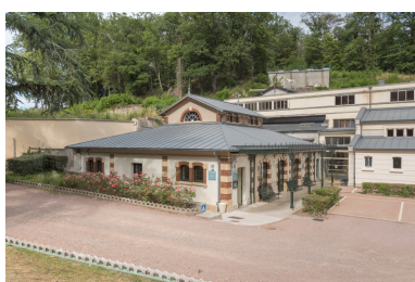
Pavillon des douches. Phot. Pierre-Marie Barbe-Richaud IVR26_20195800411NUC4A
