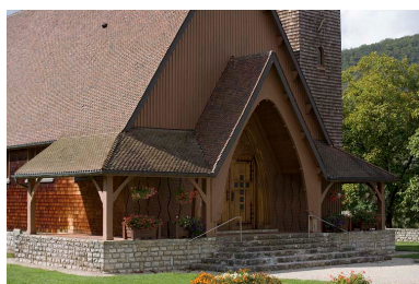
Porche. Phot. Yves Sancey IVR43_20063900087NUCA
