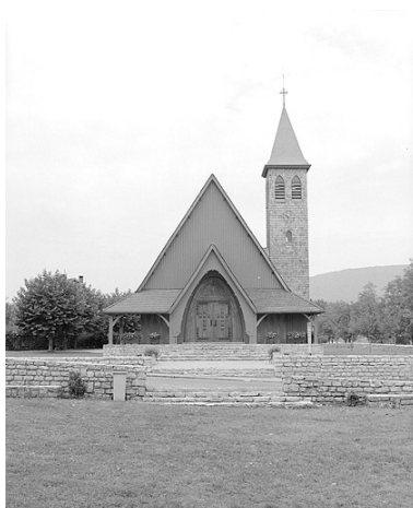
Façade ouest. Phot. Yves Sancey IVR43_19963900834X
