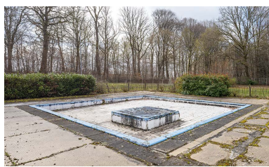
La pataugeoire extérieure. Phot. Aline Thomas IVR43_20267000049NUC4A
