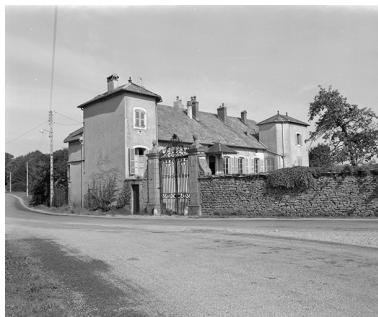
Vue de situation. Phot. Yves Sancey IVR43_19793900081X
