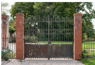
"Château neuf" : grille. Phot. Pierre-Marie Barbe-Richaud IVR26_20222100903NUC4A
