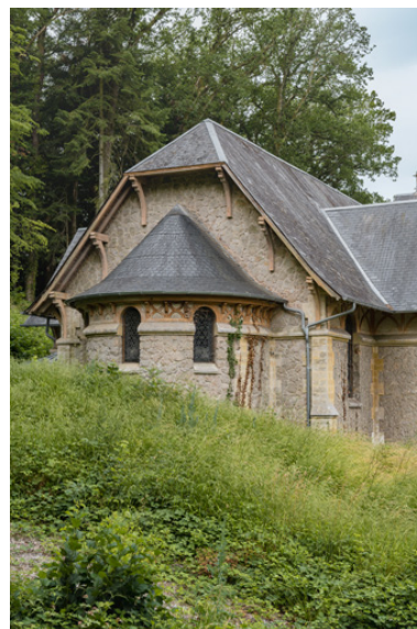
Chevet. Phot. Pierre-Marie Barbe-Richaud IVR26_20195800284NUC4A
