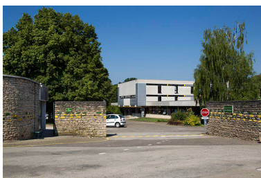
Entrée principale. Phot. Sonia Dourlot IVR43_20142500917NUC2A
