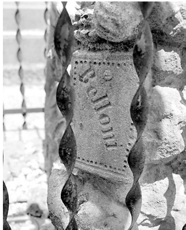
Cartouche portant la signature Belloni. Phot. Yves Sancey IVR43_20033901090X
