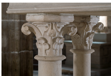
Les chapiteaux supportant la table. Phot. Nicolas Waltefaugle IVR26_20268900376NUC4A
